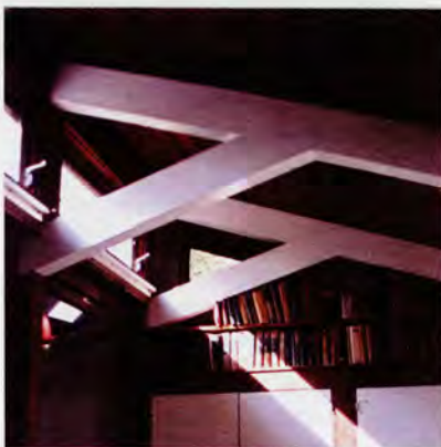
6. Scoppettone House , 1952. Interior view of trusses. Photograph by Sharon Suchma
