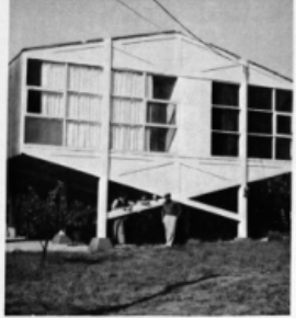
Theodore Stern House, East Marion, Long Island, 1961. "I had been looking at a book on bridges and decided to make a house with trusses. The structure elements are painted white to separate them clearly from the paneling, which is yellow. The three wall panels are red, white, and blue."
